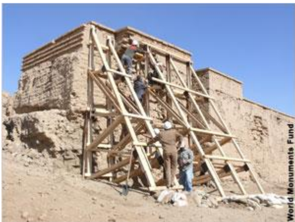
Iraqi workers shore up a fragile section of the inner-city wall as part of the World Monuments Fund preservation project.
